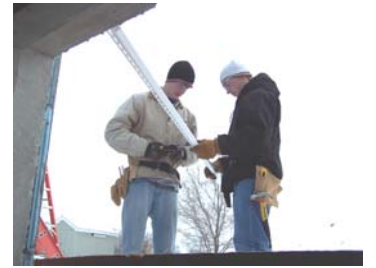
Above, Sam Kelly and Jordan Moan cut the J-channel in the back of the home. Below, Jeff Strong and Austin Nelson install the soffit. Weather doesn't stop work on the house, unless the wind chill is below 0° F.
